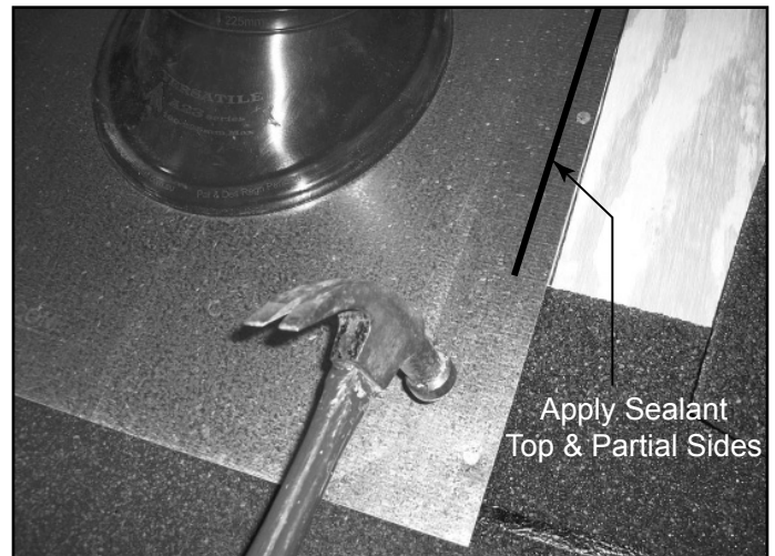
Figure 10.22 Slide Flashing Down, Secure & Apply Sealant
